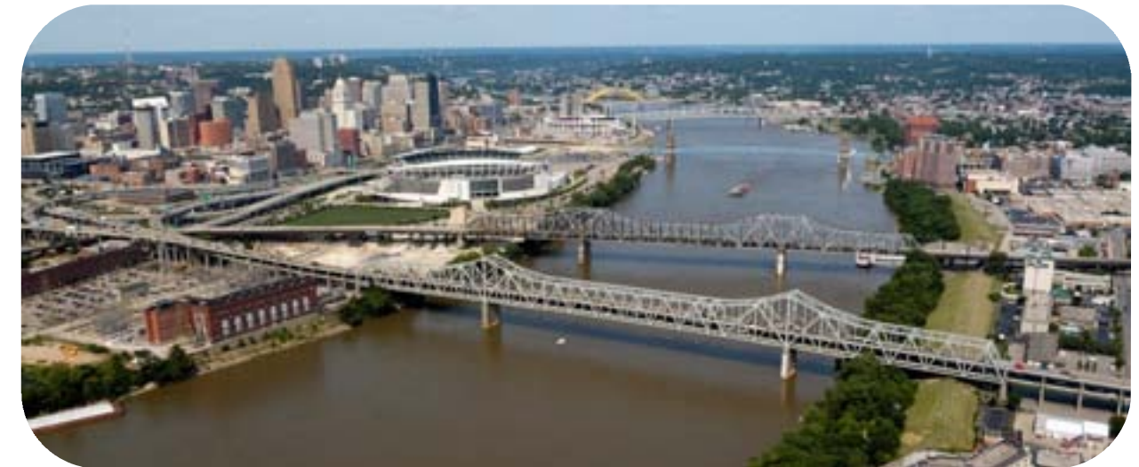
Existing Brent Spence Bridge in Forefront
